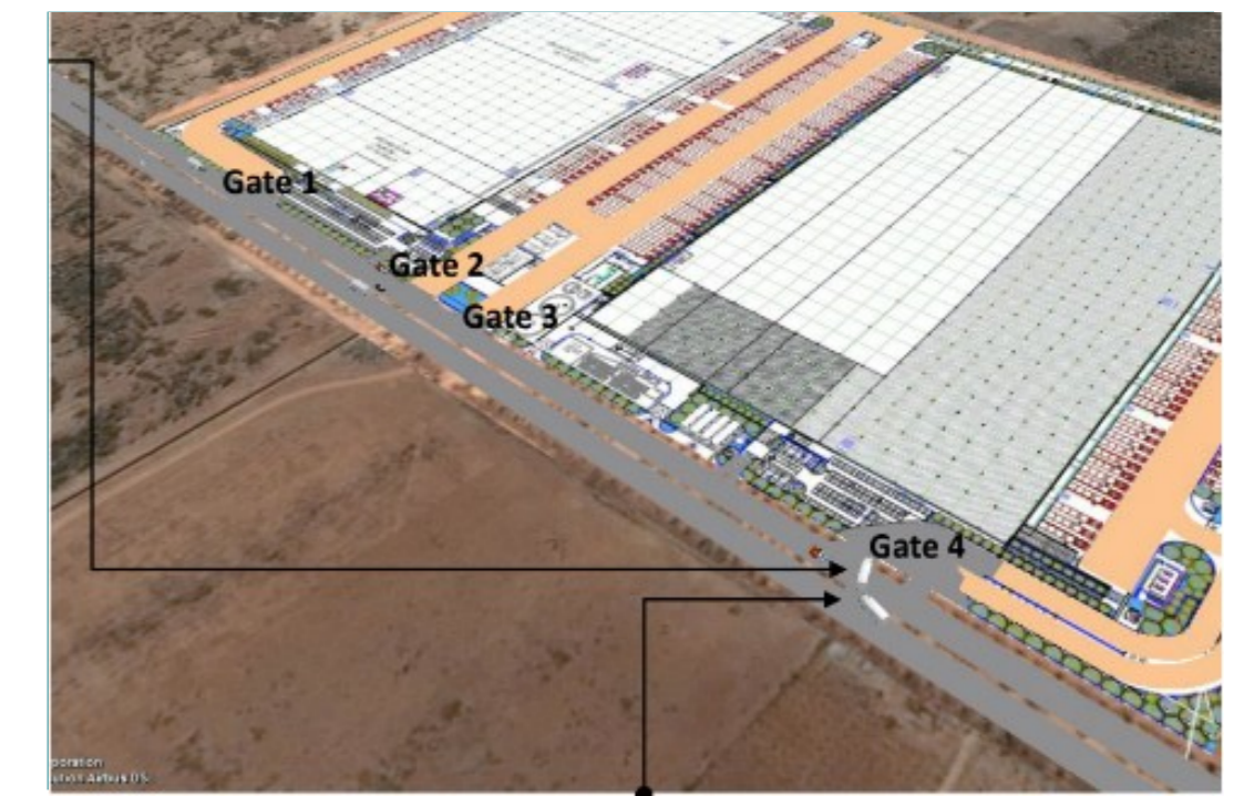
Integrated Warehouse, Amazon, Bangalore | Gurgaon
